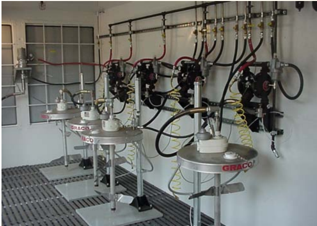
Paint kitchen installation in indoor moveable hazardous storage building
